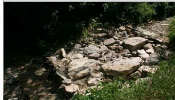
24 – Rampa in massi (29/04/2016)
