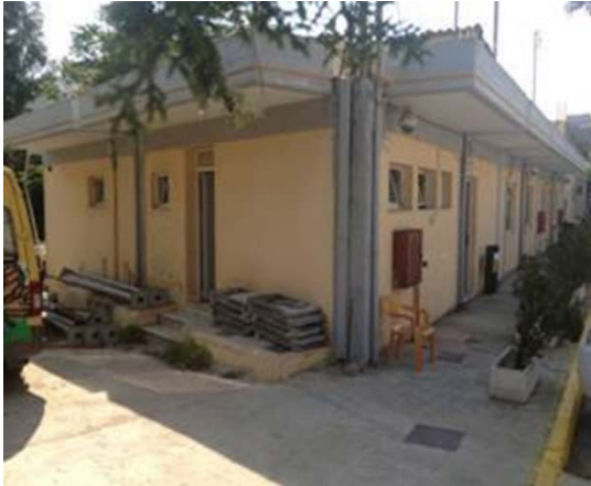
FIGURA17 – Municipal Offices (Alimos)
