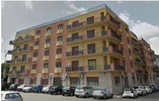
FIGURE 15 - Satellite building (Messina)
