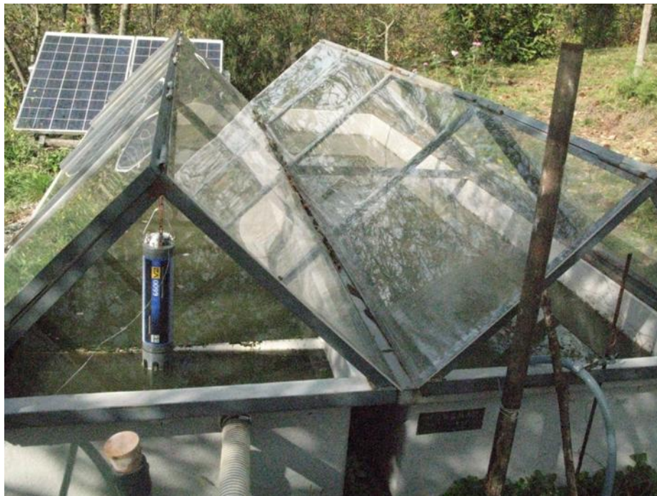
Figure 10 Phytodepuration pond placed at Le Pezze
