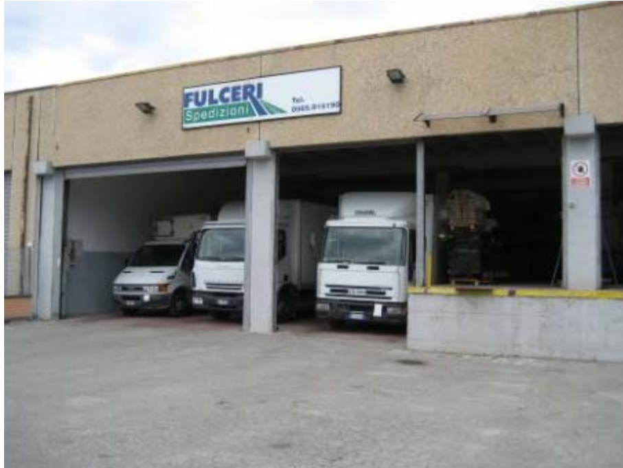
Figure 1. Logistics base of Corriere Fulceri in Portoferraio (outside view)
