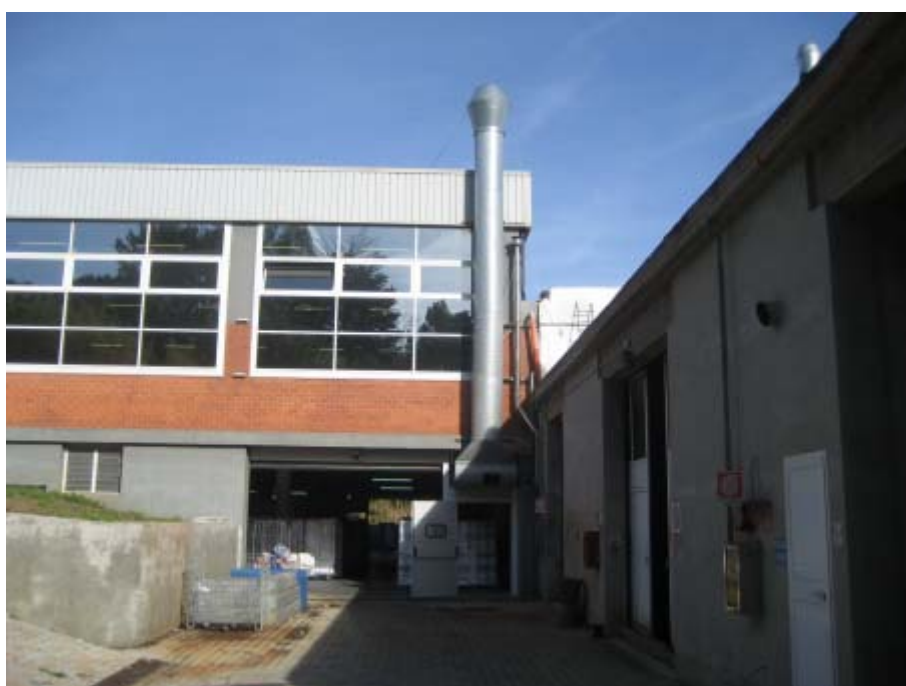
Figure 3. Premises of Lavanderia Industriale Ilva in Rio Marina (outside view)
