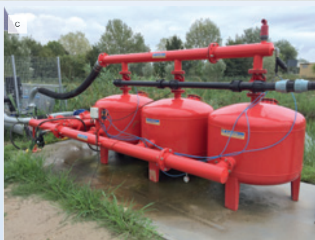
Photo 7. Small water collecting basin: (a) overview; (b) irrigation pump; (c) filter.
