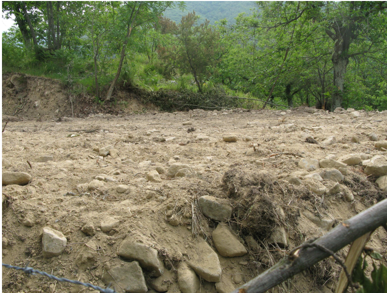
Fig.9: the levelled area available to the phytodepuration system installation
