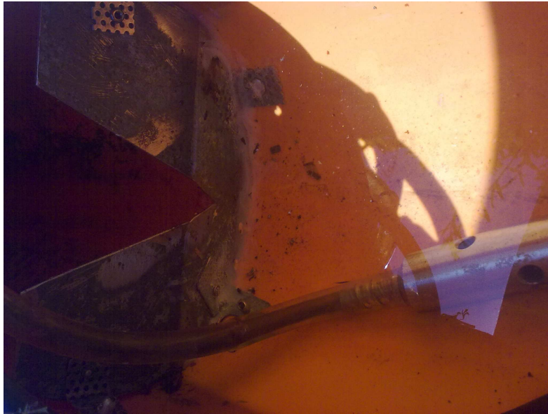
Fig. 17: particular of the triangular weir for the continuous measure of the flow into the storm water tank
