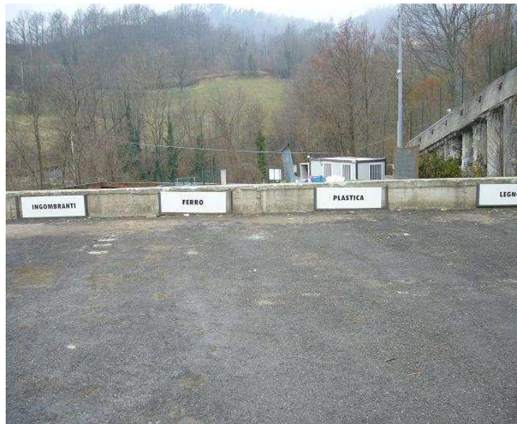
Fig. 10: municipal waste Depot: general view of the monitored area
