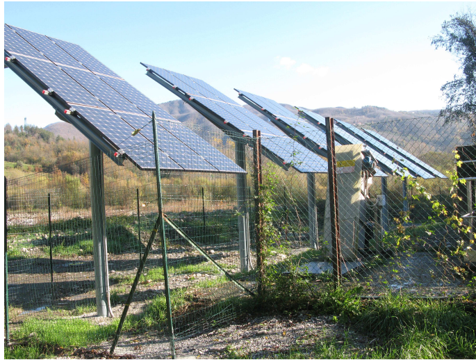
Fig. 1_b: the photovoltaic system for energy recovery built up in the selected area for the photobioreactor installation
